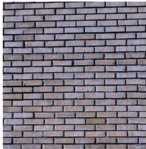
Fig 3: The original wall.
